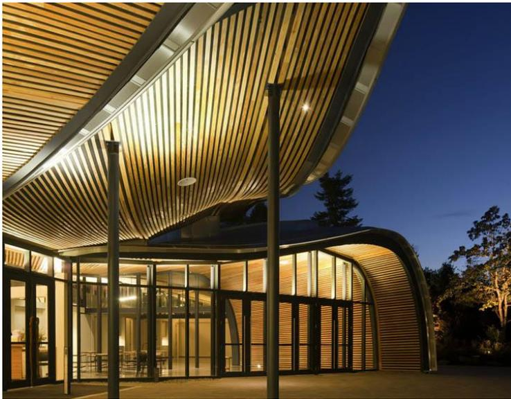
The Centre’s complex petal roof structure utilizes a glulam post and beam assembly. The beams are spanned with secondarily curved joists suspending a lengthwise fir plywood slat exposed ceiling. The assembly is topped with two layers of plywood and conceals all MEP services.
