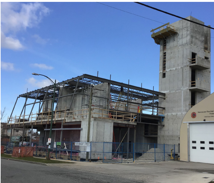
Fire Hall No. 17 construction site (Credit: HCMA)
