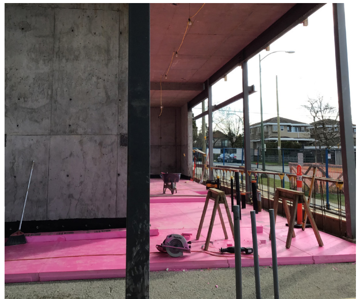
Slab on grade insulation installation (Credit: HCMA)
