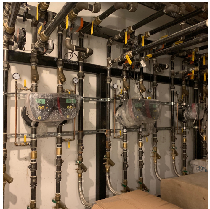
Ground source heat pump system installation (Credit: HCMA)
