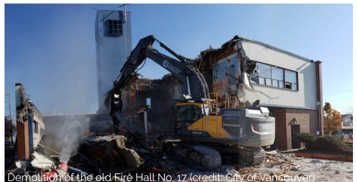
Demolition of the old Fire Hall No. 17 (credit: City of Vancouver)
