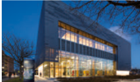
Campus Energy Center (CEC) Infrastructure (utility) – UBC Vancouver Mass timber hybrid structure
