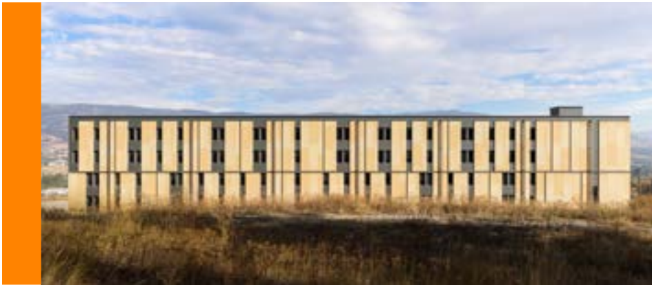
The University of British Columbia's Skeena Residence utilizes a simple building form to meet the Passive House standard. Photo credit Andrew Latreille.
