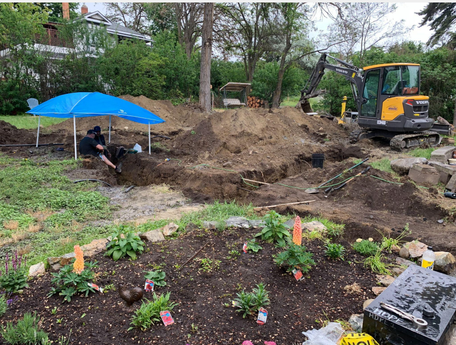
During Loop Installation
