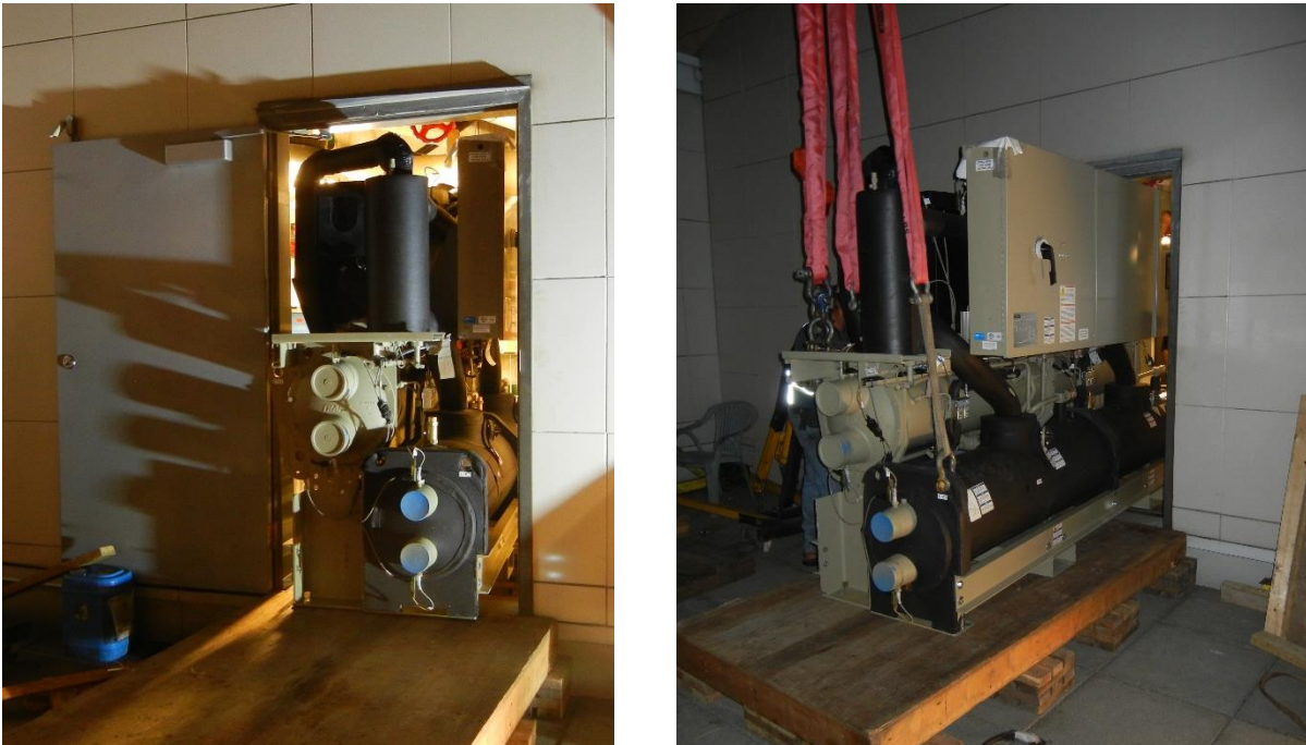
FIGURE 6: MOVING EQUIPMENT IN CONSTRAINED SPACES
